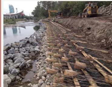
Live cribwall Couri, D., 2018
