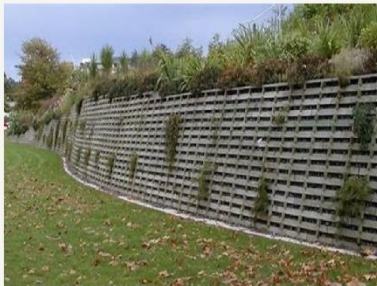
Live cribwall Hartono, 2018
