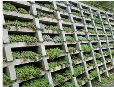
Live cribwall Bellingham Green Roofs
