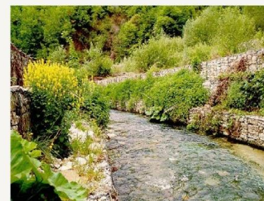
Vegetated Gabion Vegetated gabions in riverbank embankment at SP32 in Son La Province after one year and two flood seasons - ICEM, 2017
