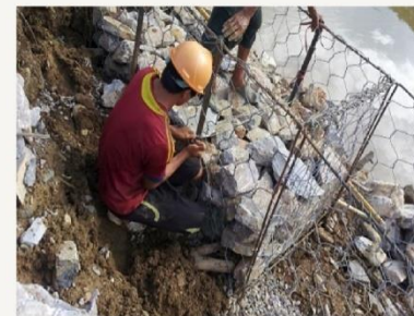
Vegetated Gabion Installation of vegetated gabions in river embankment in Son La Province - ICEM, 2017
